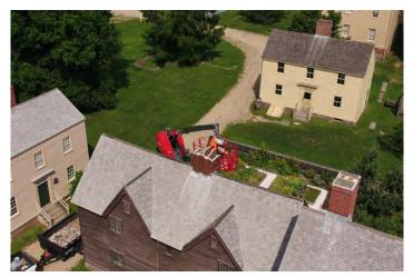
The painstaking work of removing the Sherburne House chimney that was built in the 1960s and had deteriorated beyond the point of repair. (Credit: David J. Murray/ClearEyePhoto.com)
